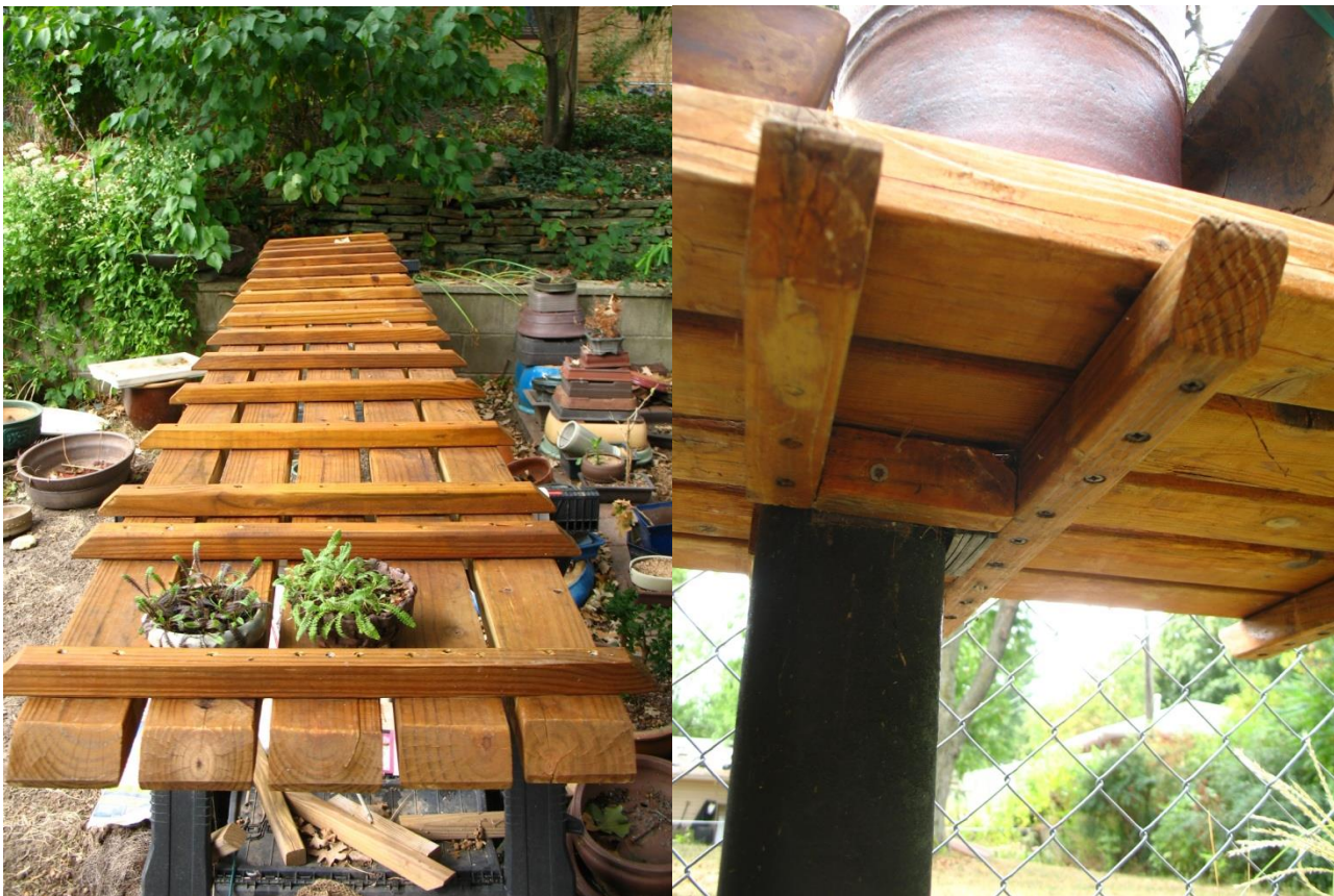
New 12' x 22" bench under construction; bottom.
